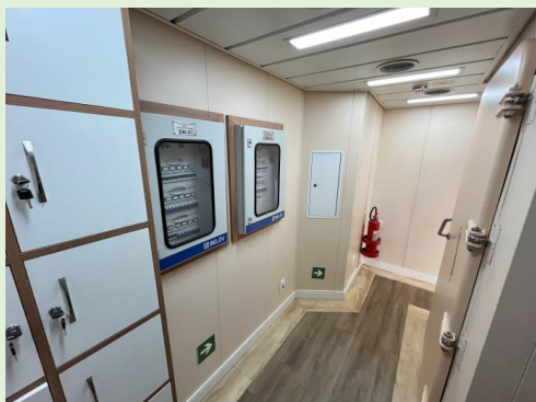
Corridor Stern Deck
