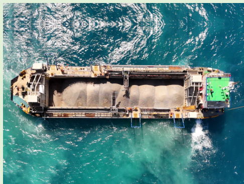
Top View Operation Site
